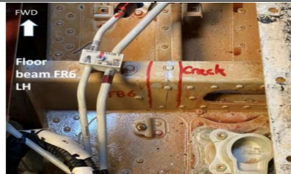
Figure 11: LH Floor beam at Frame 6
